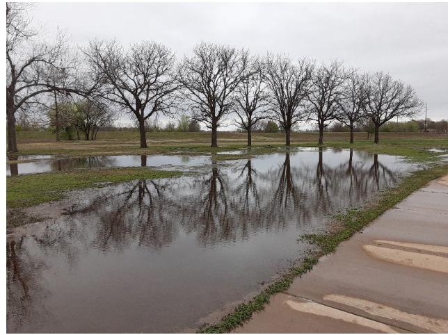
Figure 1. A landscape area with a significant ponding problem. Appropriate alternatives for this significant ponding problem, with existing large trees are discussed in drainage problem 1.
