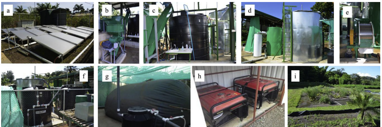
Fig. 2. The pilot system at Fabio Baudrit Agricultural Station a. Solar thermal collectors, b. Grinder, c. Feeding tank, d. Thermophilic CSTR and hot water tank, e. Liquid and solid separator, f. Liquid effluent tank, g. Biogas bag, h. Engines, i. VFSS-CTW.
