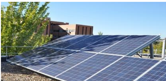
Figure 8: Shadow cast every day on Array 2 by a tree located at its west.
