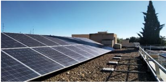
Figure 7: Shadow cast every day on Array 2 by a tree located at its east.
