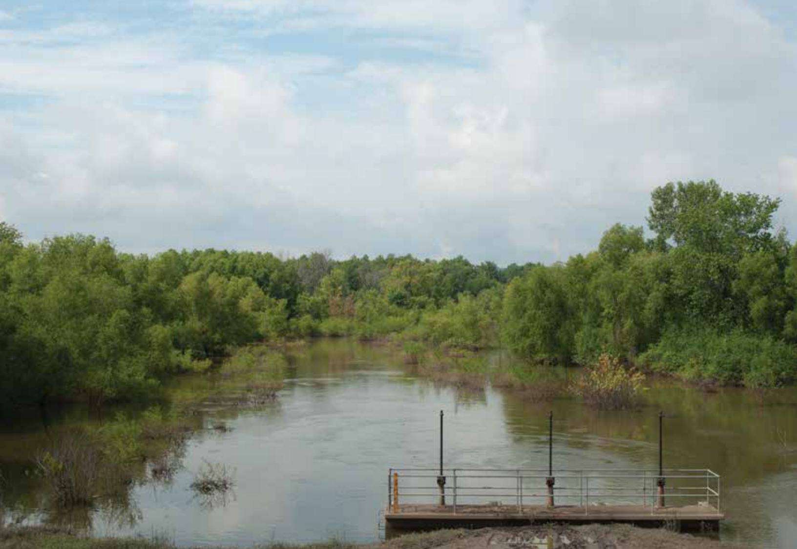
Lock at the mouth of the culvert in the levee at the Fountain Creek Pump Station during the 2011 flood
