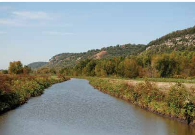
Fults Creek Diversion Ditch
