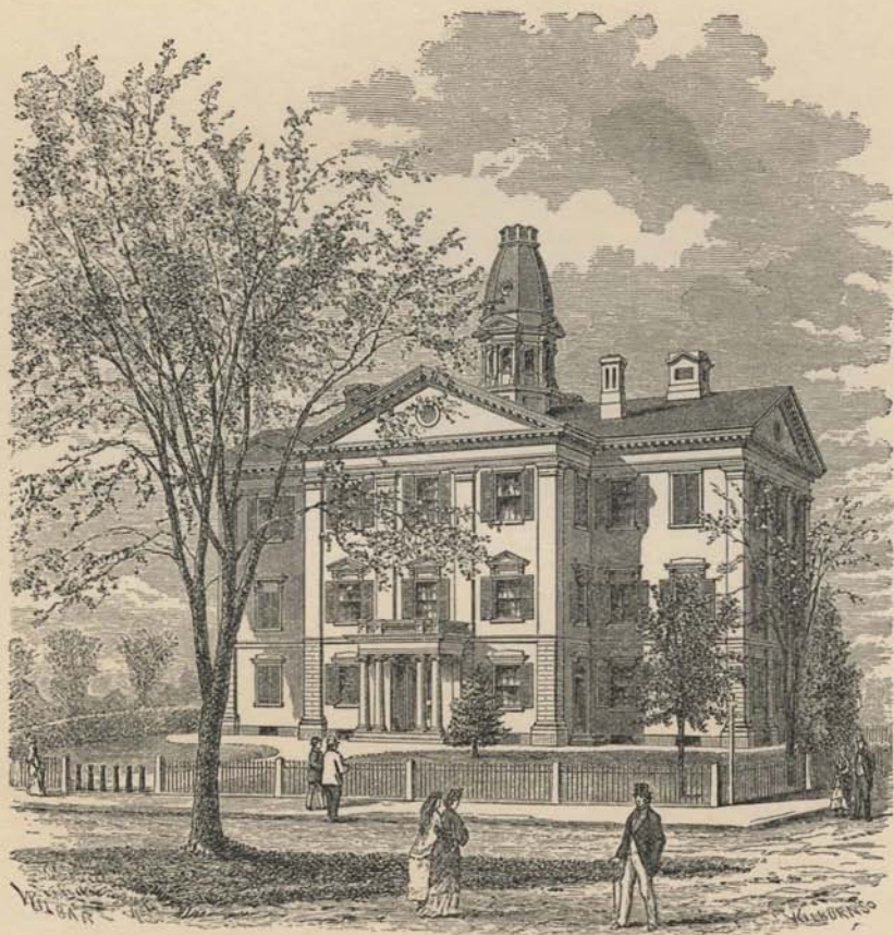
The Second Enlargement of the School Building in 1871, by adding a story sixteen feet in height, with Observatory on the centre.
