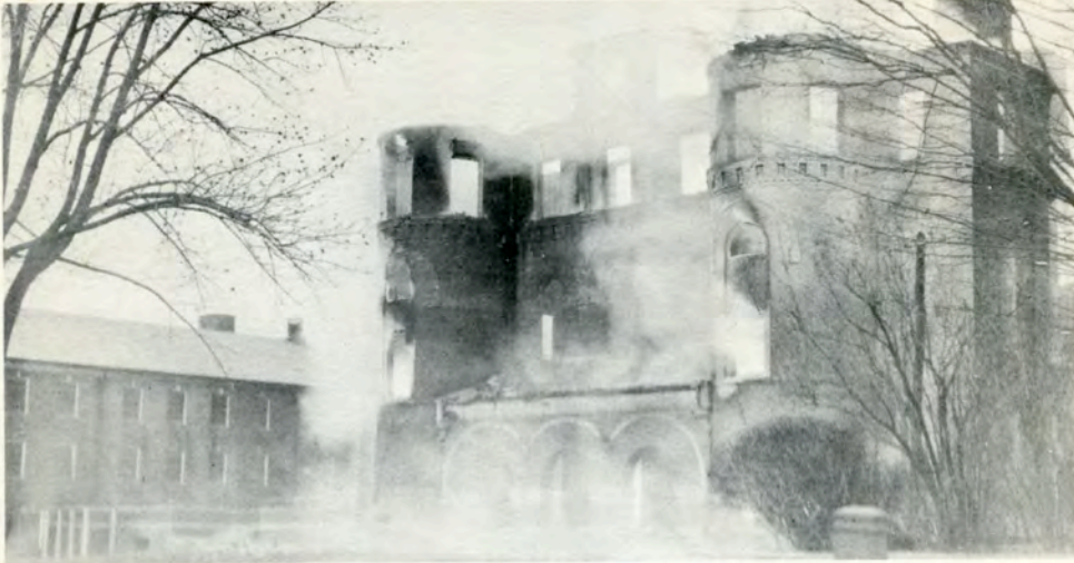
The still smouldering hulk of what had once been the handsome brick Normal School.
