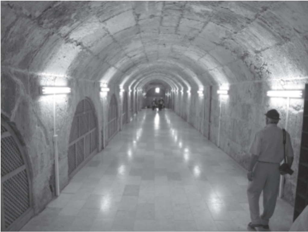
Figure 4: Vaulting of the western most vaulted passage of the Triple Gate. Source: Awwad, 2013
