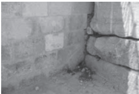
Figure 11: Detail of the portal from the north showing beginning of the 8th arch. Source: Awwad, 2012.
