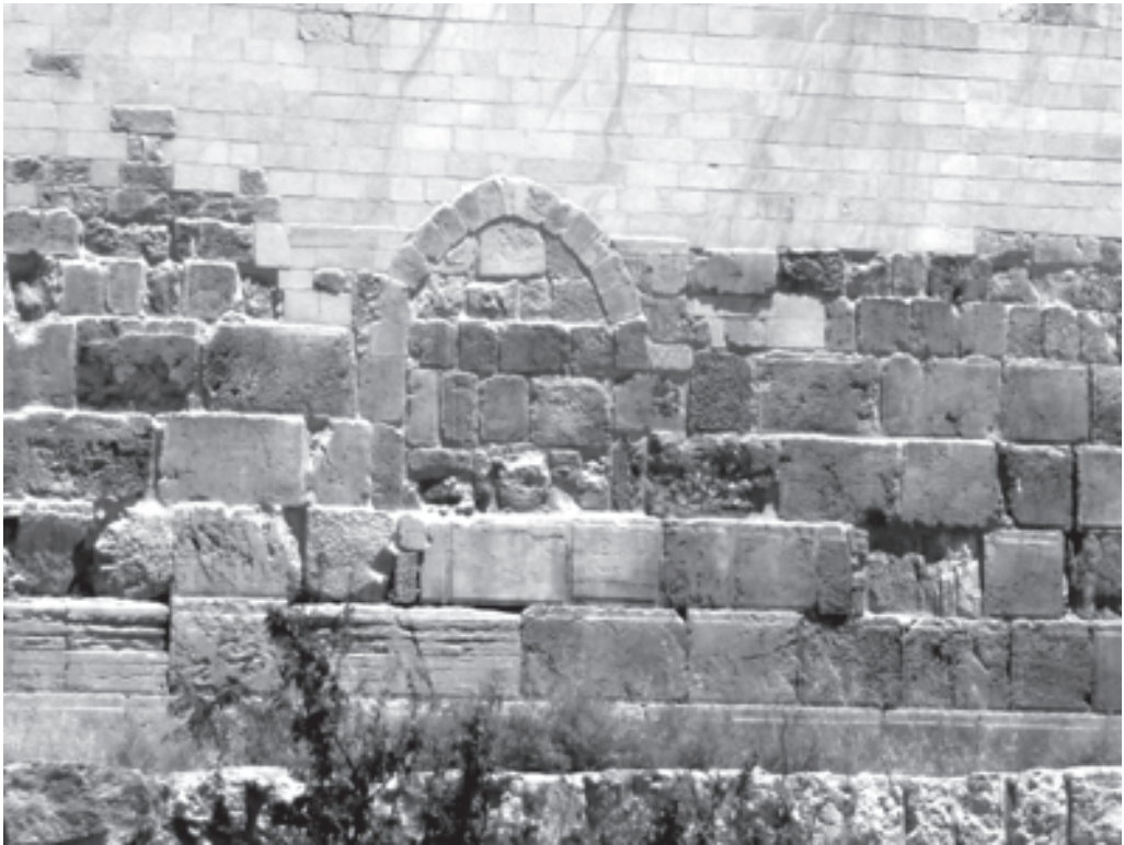
Figure 9: Single Gate in the southern wall of the Haram al-Sharif located east of the Triple gate. Source: St. Laurent, 2012.
