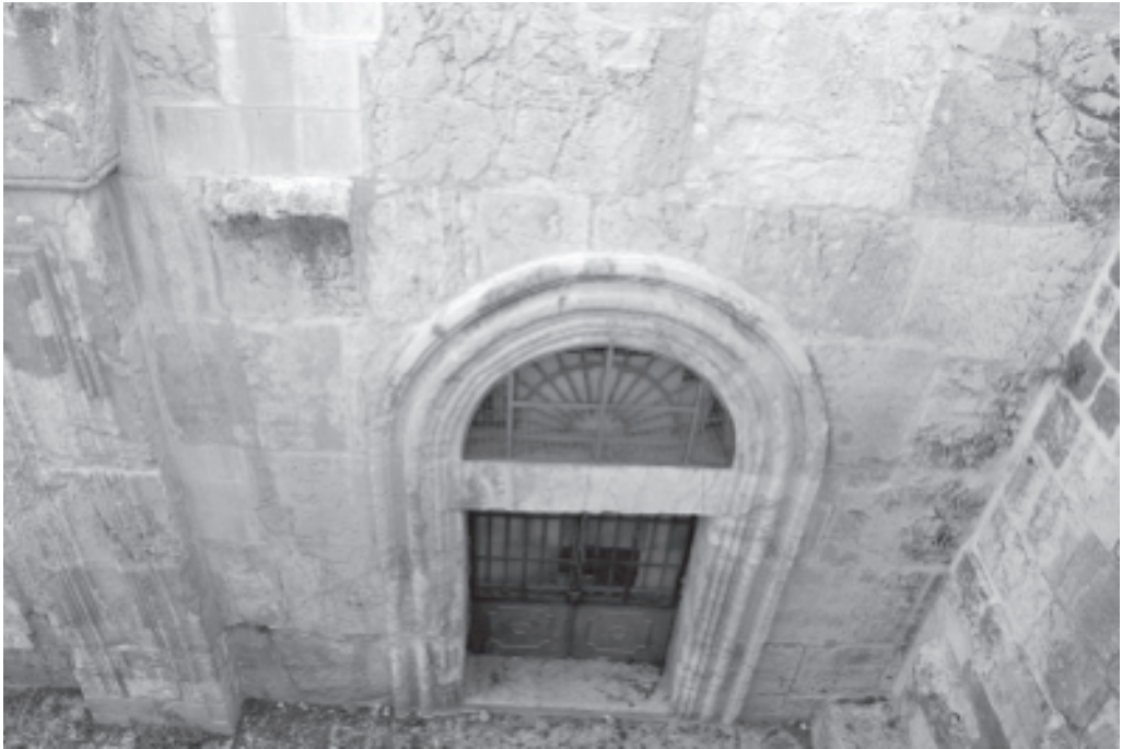
Figure 15: South entrance of the Golden Gate from the south. Detail shows the springing of an arch to the upper left of the entrance. Source: St. Laurent, 1993.
