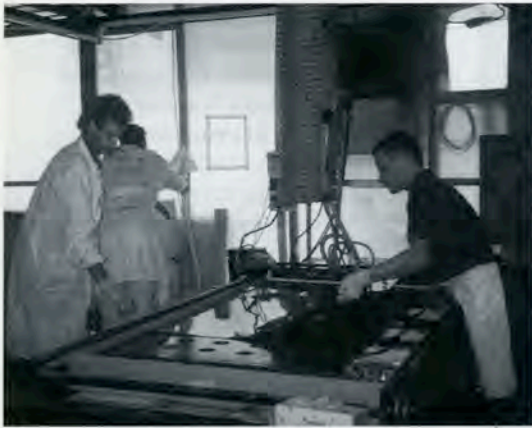
MIVAN, a Belfast Irish firm, produced gold panels. The workshop was on site beside the Dome of the Rock. This photo shows the pressure plating of 2 micron thickness of gold held in emulsion to panels which had already been plated with copper and nickel. Computer regulated quality control of the thickness of gold took place in an adjoining room.
