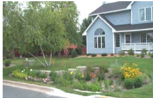
A raingarden installed as a LID technique to treat residential runoff.
