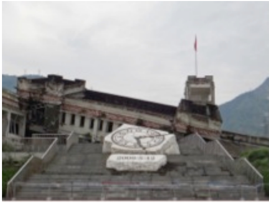
Figure 14 A Huge Broken Clock in Xuankou Middle School Ruins in Yinxiu Town 66
