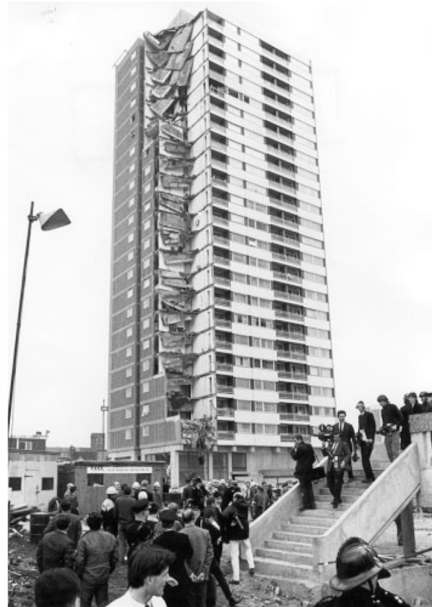
Figure 1-2 Ronan Point after collapse (Pearson and Delatte, 2005)
