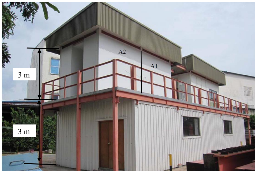
Fig. 3.1 Photo of monitoring station
