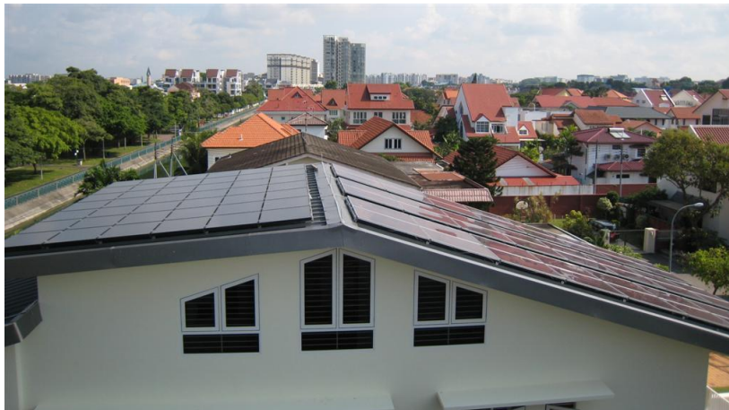
Fig. 6.1 The first zero energy house in Singapore.
