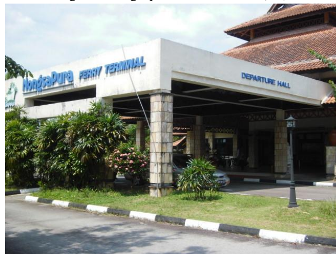
Fig 3.3: Nongsapura Port in Batam (R2)
