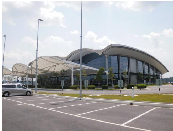
Fig 3.2: Puteri Harbour Port in the Johor State (J6)
