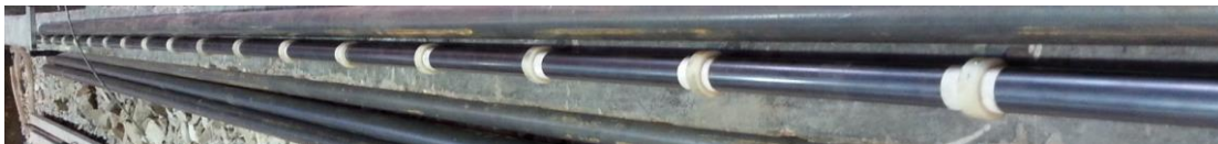
Figure 7-2 Spacers installed on the inner pipe
