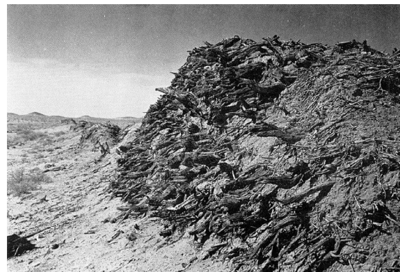
Fig. 4 XiXia long wall in Mongolia (section build of saxaul) (photo by T. Baasan in 1970s)
