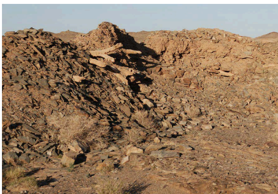
Fig. 13. The wall of the Chingisiin Khar Khot fortress made of cobblestone, earth and wood
