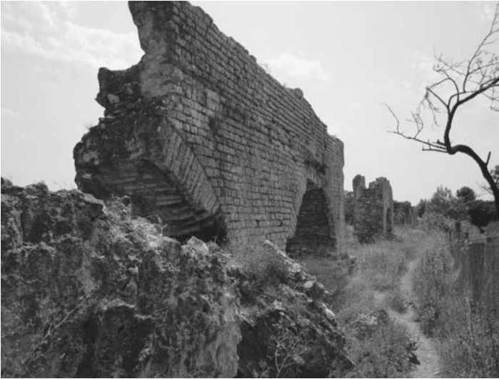
Figure 1.3 Some leftovers of a Roman aqueduct near Fontvieille, France.
