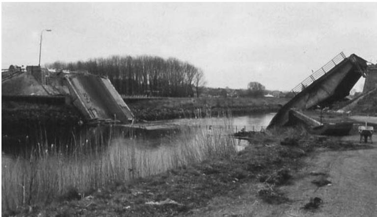
Figure 2.1 Collapse of the Melle Bridge, Belgium, 1991.
