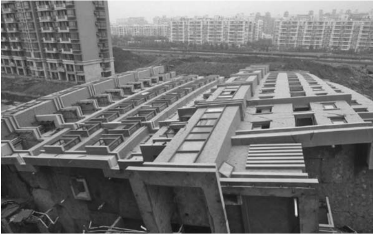
Figure 2.5 Tumbling collapse of apartment building in Shanghai, 2009 (Internet photo).
