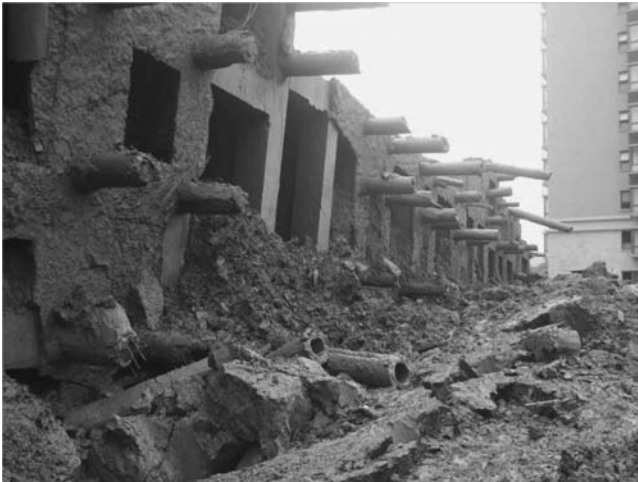
Figure 2.6 Detail of the foundation piles (Internet photo).
