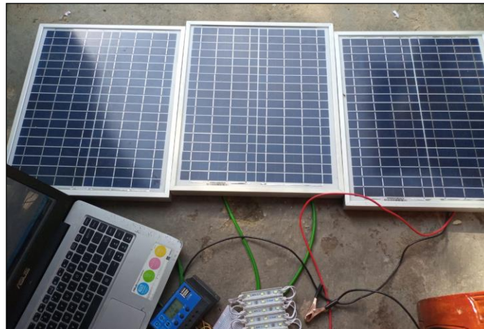
Figure 3. Calibration of solar panel conducted
