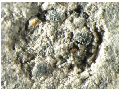
Fig. 6. S-6-Middle-3: Voids filled with crystalline material
