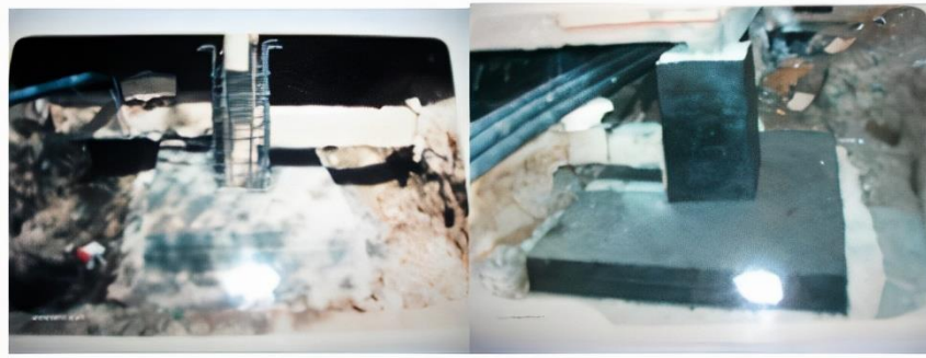
Fig. 10. Foundation and primer columns after repairation
