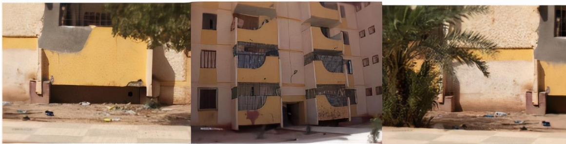
Fig. 11. Building after repairation
