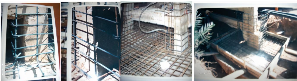
Fig. 9. Reinforcement of the foundations and primers columns
