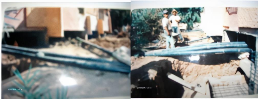
Fig. 6. New sewer lines to evacuate wastewater
