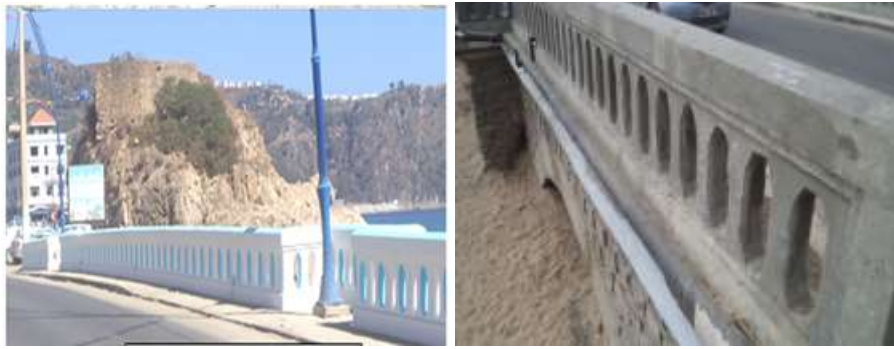
Fig 6. Bridge after rehabilitation Works.
