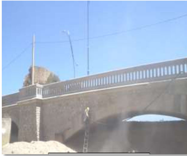
Fig 1. Elevation view of the structure
