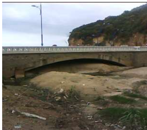
Fig 2. Bridge over the River river Kentra Stora, in Skikda.
