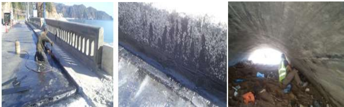
Fig 5. Bridge Repair Works.
