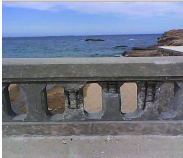
Fig 3. Defects affecting the reinforcing concrete.
