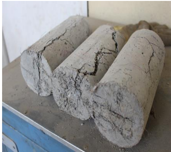
Fig 8. Test for Splitting Tensile Strength of Concrete
