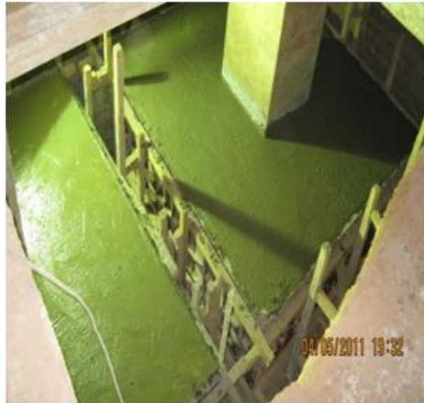
Fig 8. Fresh concrete casted in the enlarged area of the footing
