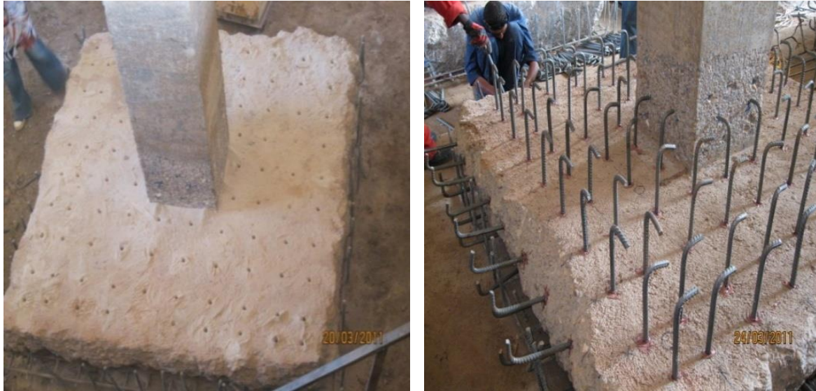
Fig 5. Drilled holes and inserted dowels bars.
