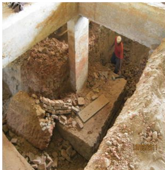
Fig 4. Excavation around the footing.
