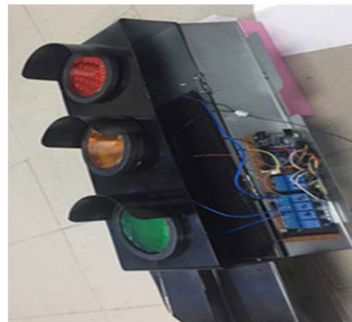
FIGURE 8. Installation of components in traffic light housing.
