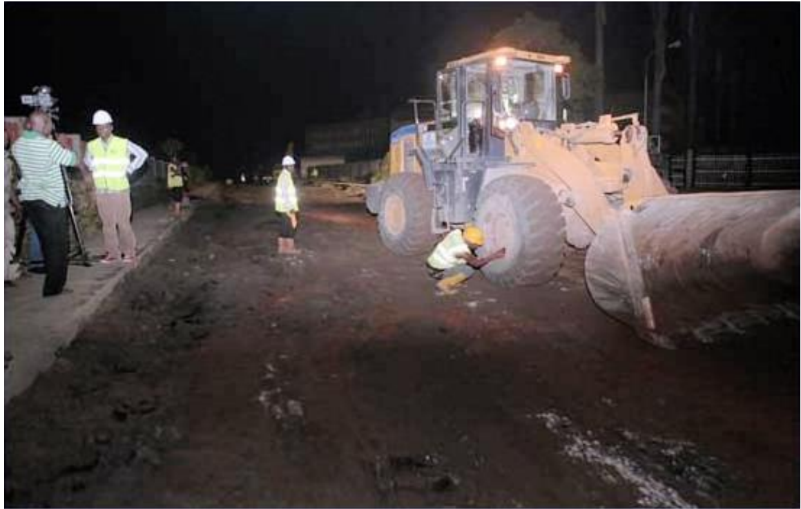
Figure 8.8: Case Study 2 project site (work being undertaken at night)
