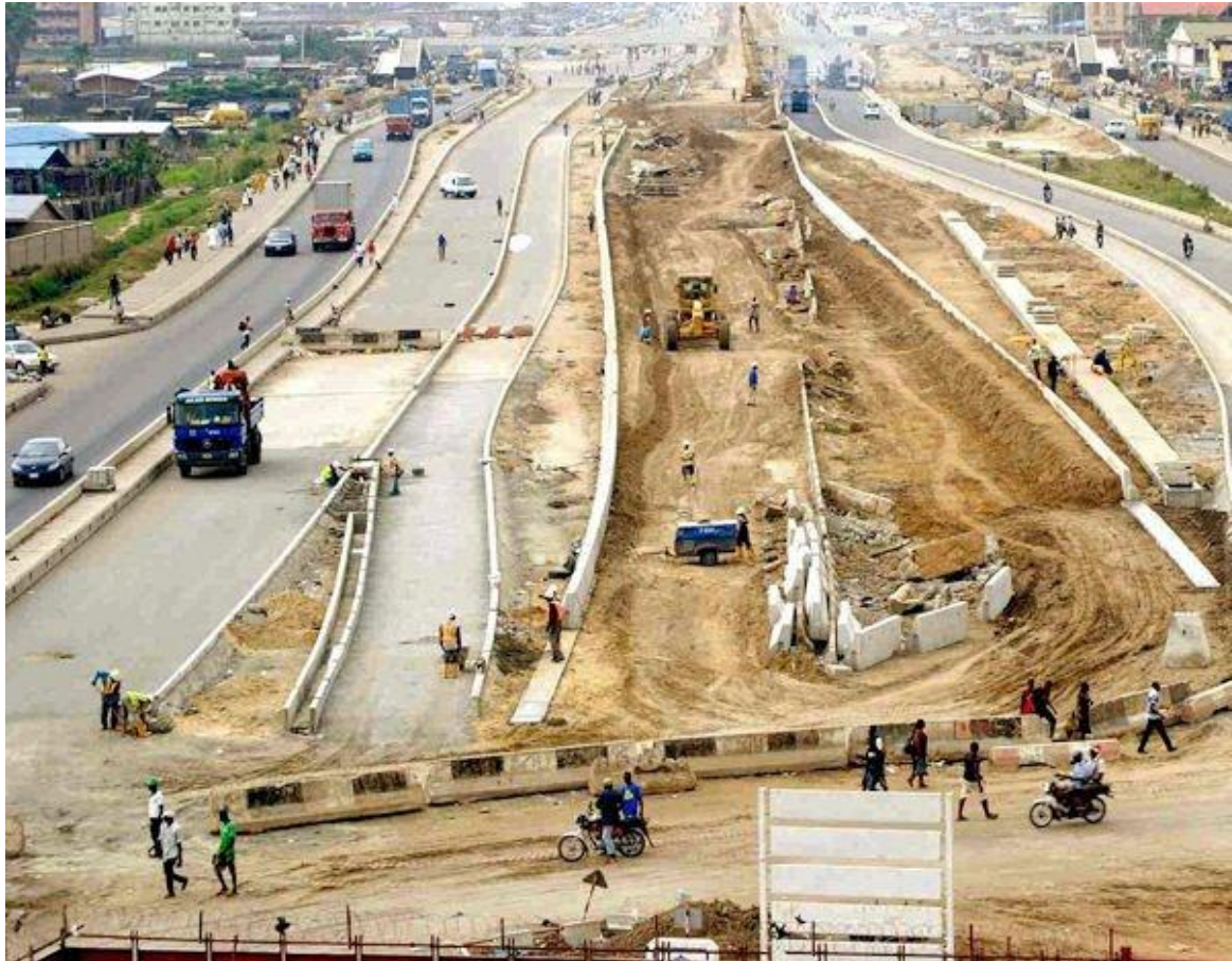
Figure 8.6: Case Study 1 project site (on-going work)
