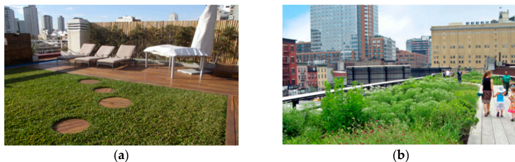
Figure 4. Semi-intensive green roofs: (a) Buenos Aires, Argentina [24]; (b) High Line park building, New York [25].
