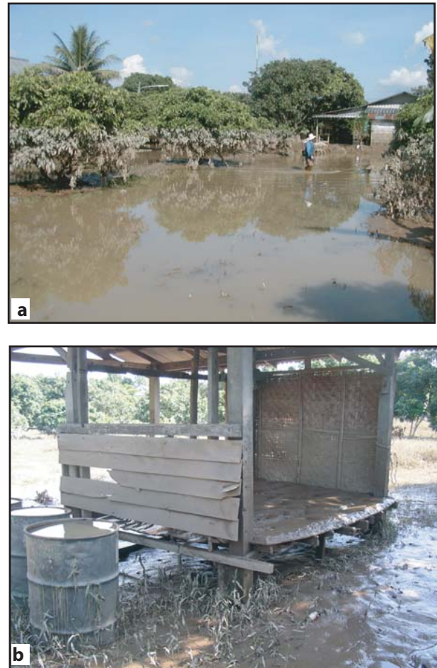
Fig. 8. (a) High water line on fruit trees. Floodwater depth was 1.3 m. Location is at point B of Fig. 11. View is to the southeast. (b) hut located at point H1 on Fig. 11. Five cm of sediment deposited on platform elevated 0.55 m above ground and 8 cm of sediment on surrounding ground (see Fig. 12). Photos taken on 2 October.
