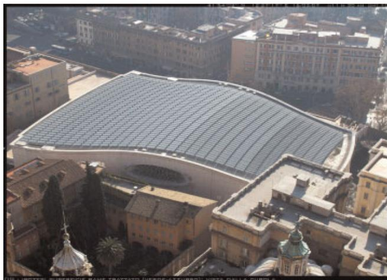
Figure 2:3 – Example of rooftop application of opaque photovoltaic modules Source: (Pagliaro et al., 2010, pp. 61)
