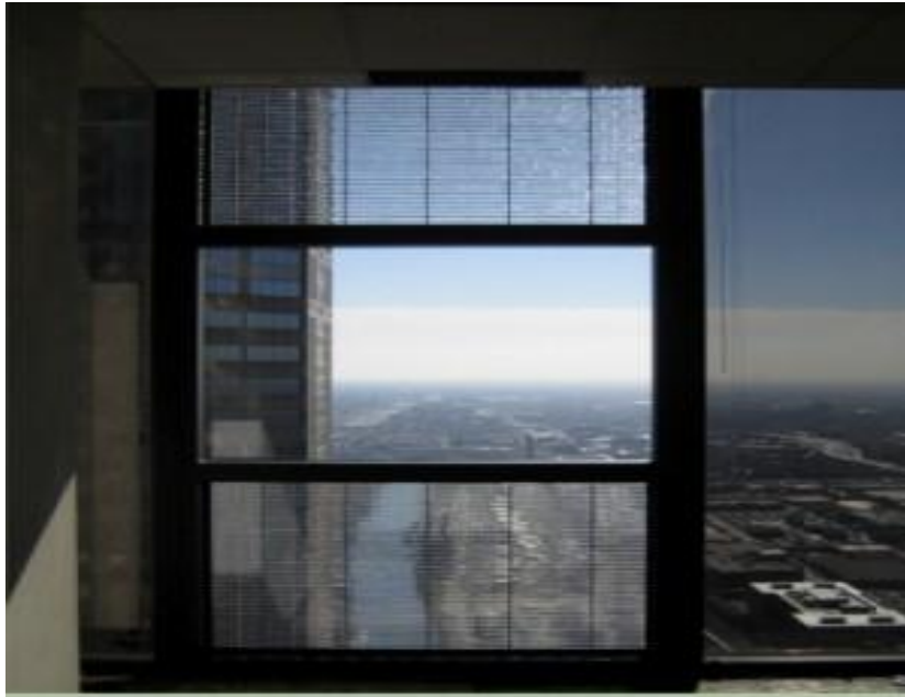
Figure 2:5 – Indoor view of a semi-transparent BIPV window
