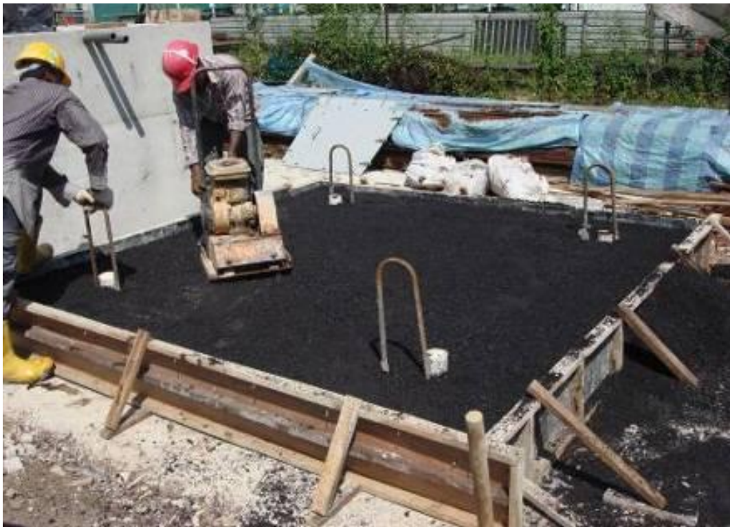
Figure 4.6 Compaction of asphalt layer
