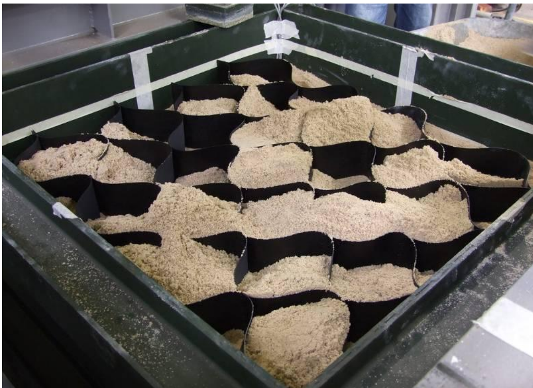
Figure 3.6 Geocell used to reinforce the sand in the steel strong box
