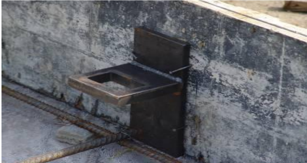
Figure 4.19 Accelerometer mount cast in-situ
