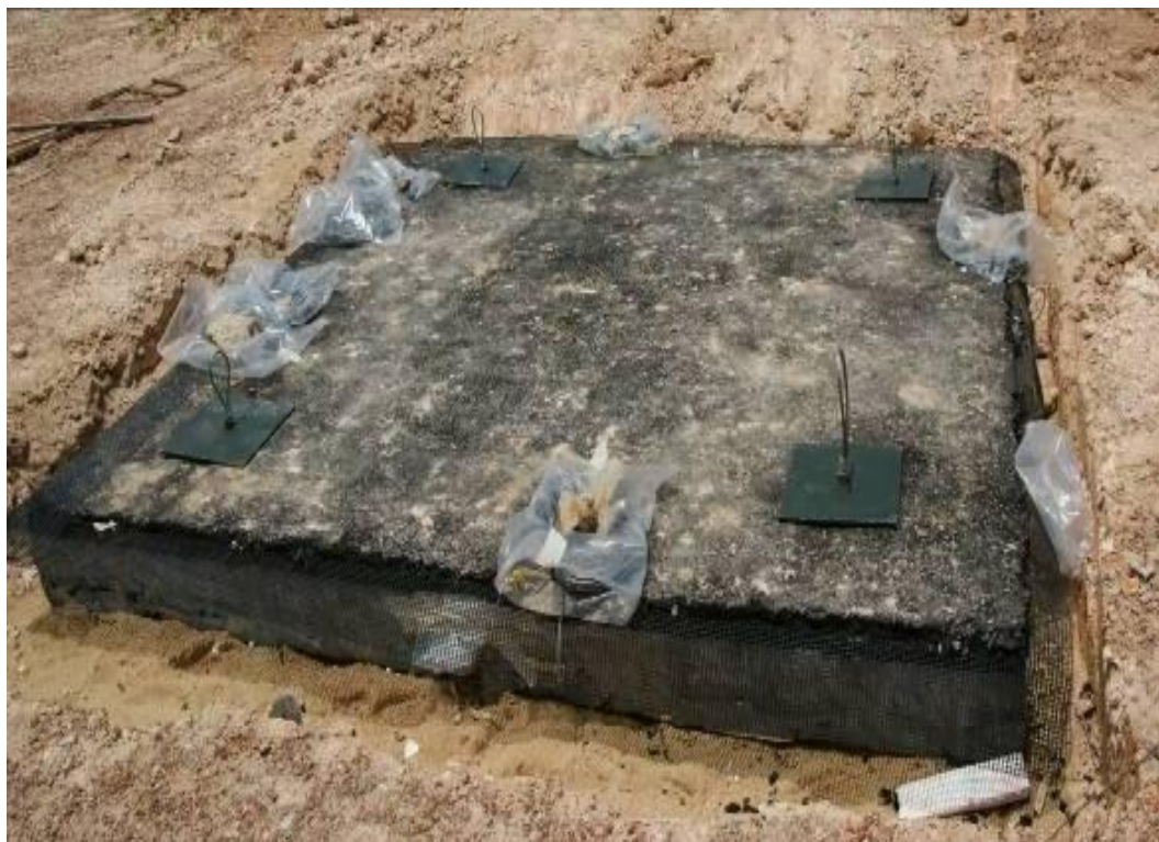
Figure 4.12 Completed Slab 2 with Anchoring at site
