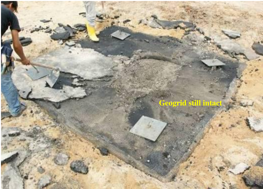
Figure 4.36 Removal of top section of asphalt for Slab 2
