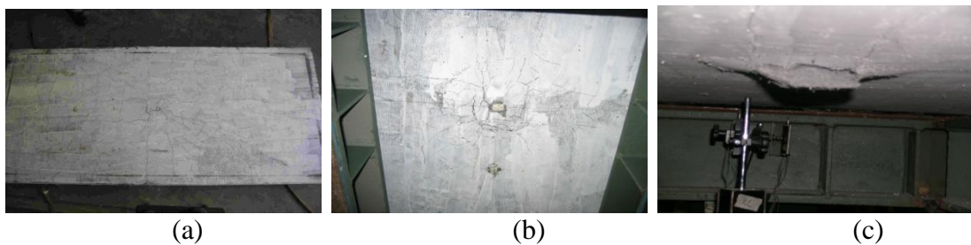
Figure 2.26 Damage development of ECC panels on distal face after 10 impacts (only very fine cracks developed, highlighted using a thick marker: (a) ECC100, (b) ECC75, and (c) ECC50 (after Zhang et al. 2005)
