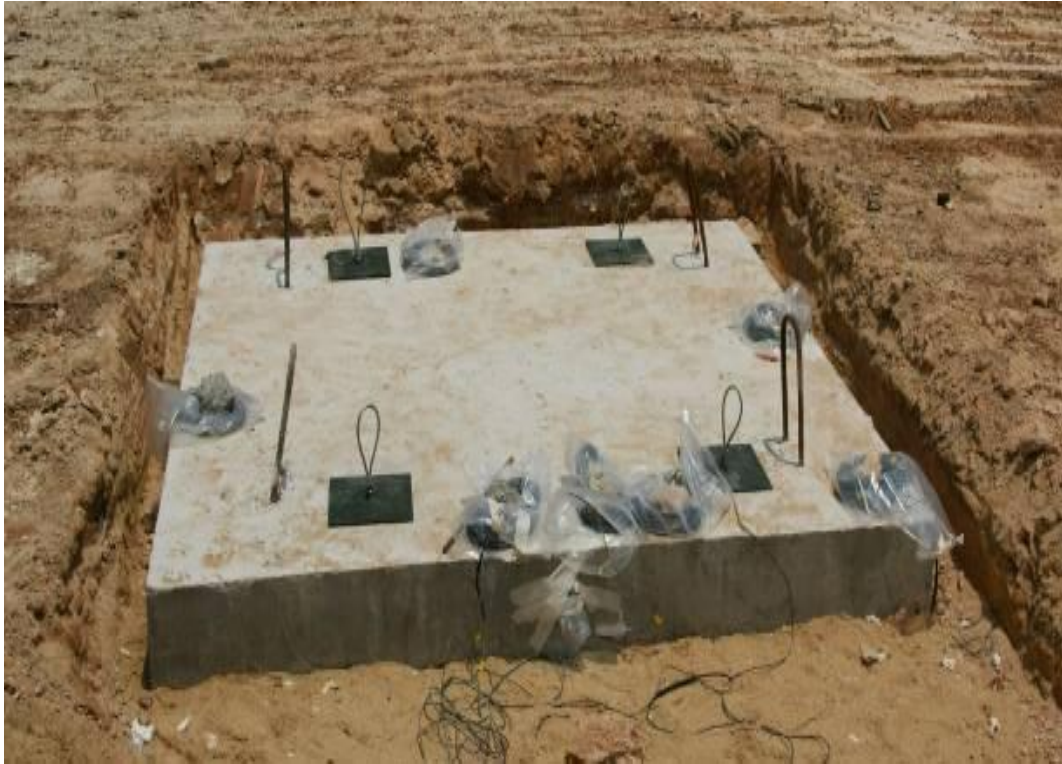
Figure 4.11 Completed Slab 1 with anchoring at site
