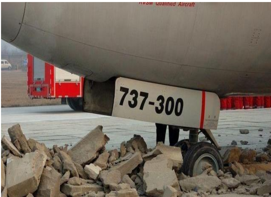
Figure 1.2 Runway was destroyed by the impact load (from http://gizmodo.com/5869715/why-did-this-airplane-landing-gear-destroy-this-concrete-runway )
