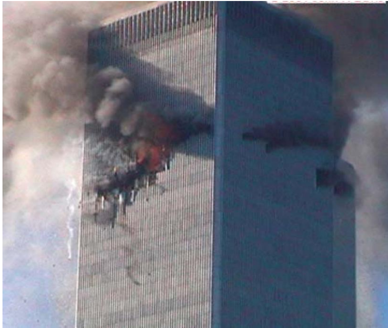
Figure 1.4: Aircraft entry hole on the north side of WTC1, 30s after impact (NIST, 2005)
