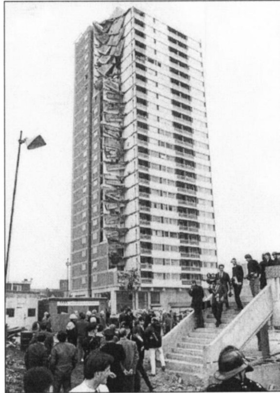
Figure 1.2: Partial collapse of Ronan Point Apartment (Griffiths et al., 1968)
