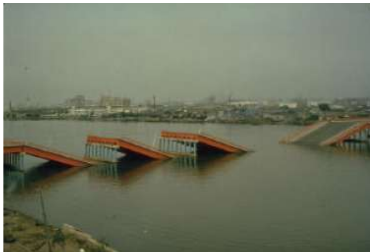
Figure 1-8 Collapse of Showa Bridge due to large lateral deformation during the 1964 Niigata Earthquake (Iwasaki, 1972b)
