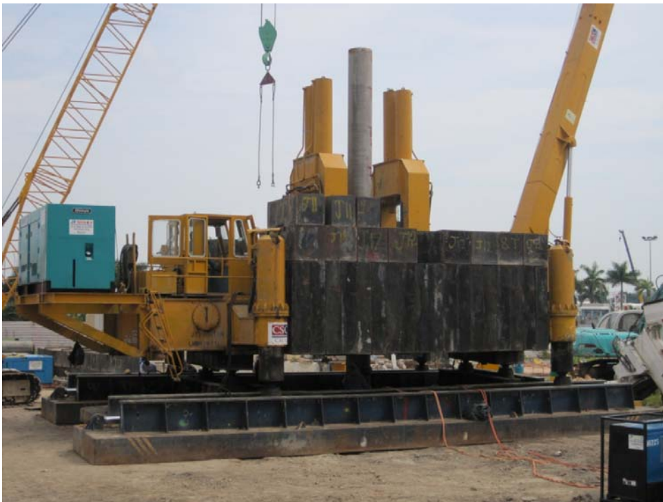
Figure 5-23 The photo of jacked-in rig used to install the test piles.
