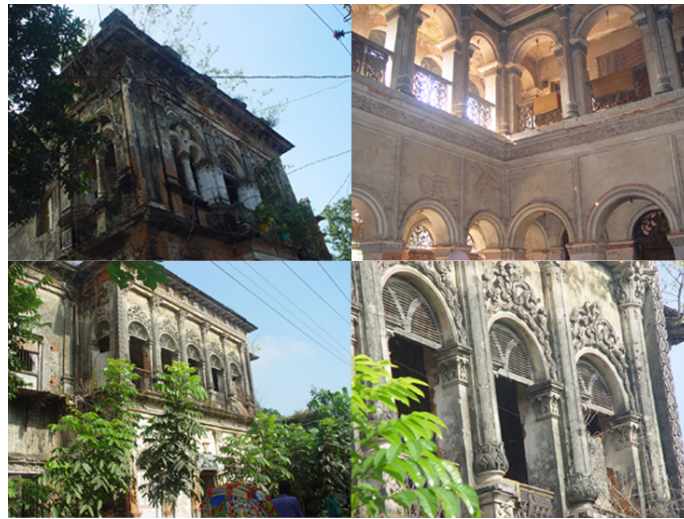
Figure 39: Heritage buildings of Panamnagar before conservation, source: author.
