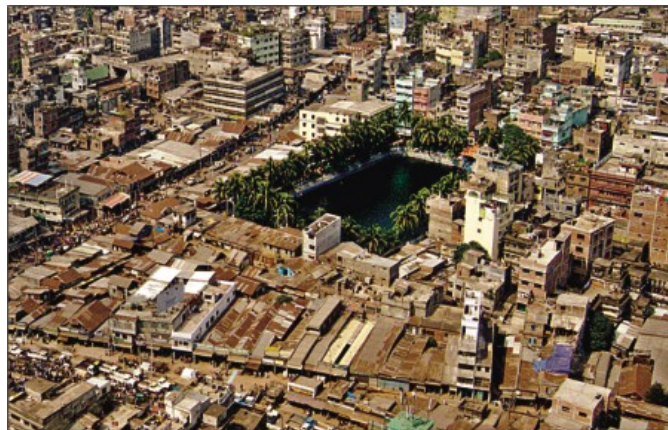
Figure 50: Aerial view of Bangshal pond, source: www.thedailystar.net/story.php?nid=31354 , accessed on 4 th December, 2010.
