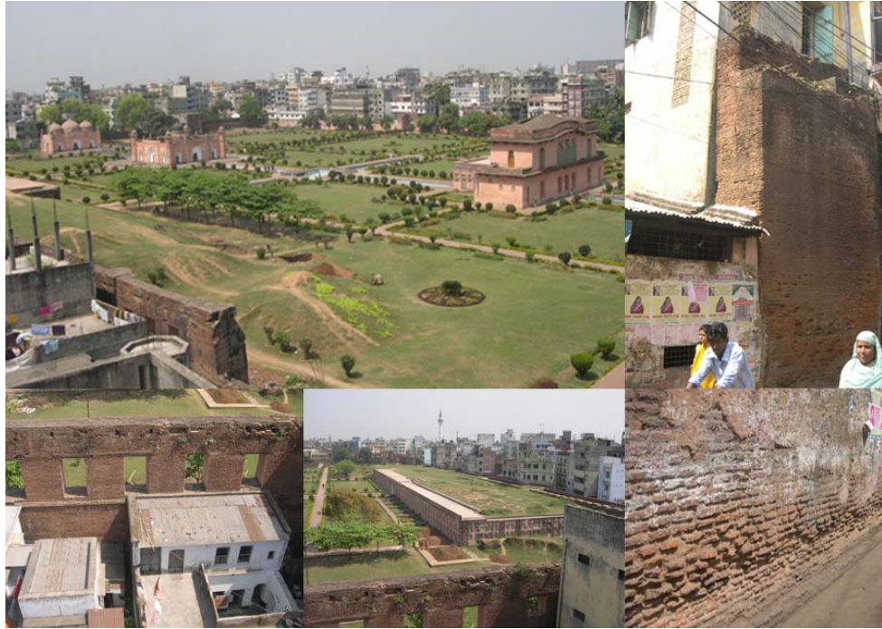
Figure 43: Illegal encroachments at Lalbag fort, source: author.
