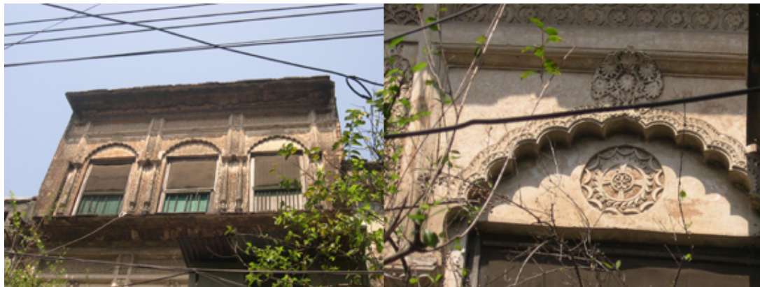
Figure 33: Stucco ornamentation in Old Dhaka, source: author.
