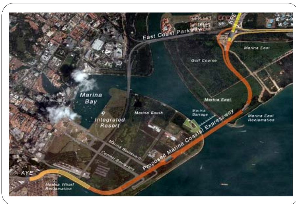
Figure 4-10: MCE road tunnel in Singapore
