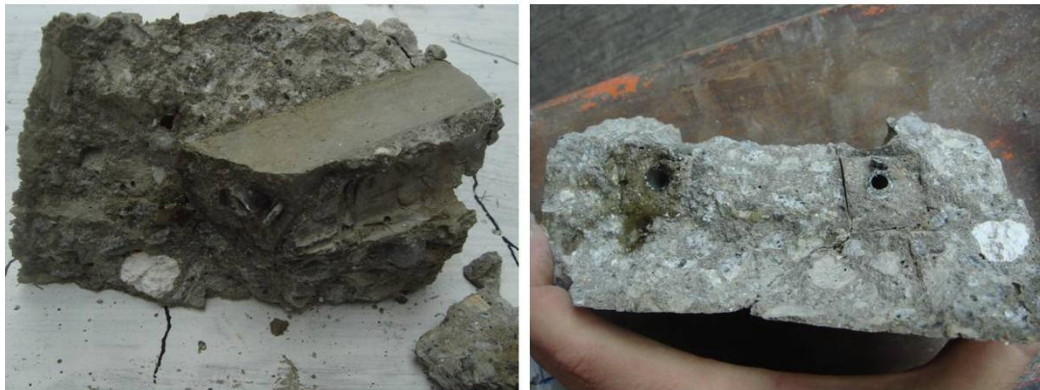
Figure 5.9: Self-healing unit protected with 6.5 strip mortar and the surrounding concrete
