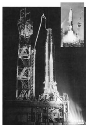
Fig A-10. Atlas missile ready for test launch. The Atlas was the U.S. Air Force's first operational ICBM. (Source: Web site of U.S. National Park Service, http://www.nps.gov/mimi/historyculture/atlas-icbm.htm )
