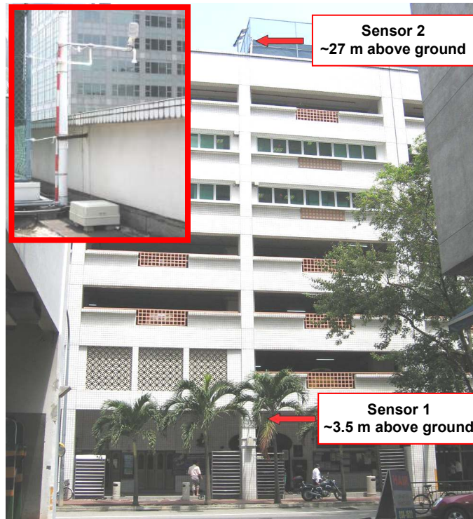
Figure 4.18: Location of canyon and rooftop sensors. Rooftop sensor inlets protrude 0.5 m away from the building wall into the canyon. Inset shows set up used for the rooftop measurement.
