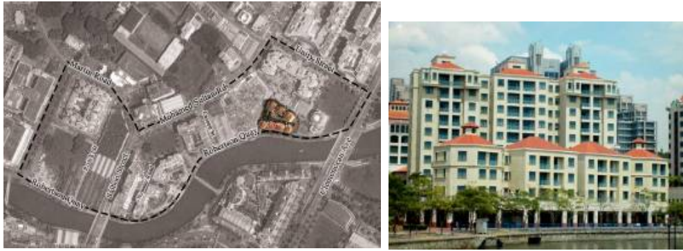
Figure 83 The Riverside View aerial picture and photo
