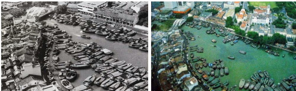
Figure 13 Left , picture of Boat Quay in 1800; right , Boat Quay in the 1980s after river cleaning.
