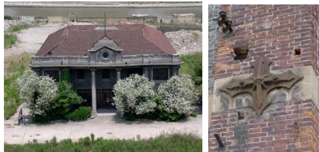
Figure 130 The office building of Fufeng Flour Factory and the façade details
