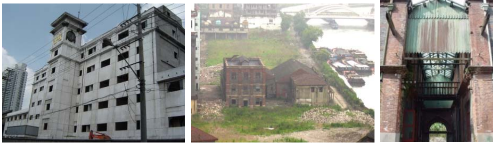
Figure 129 Left , No.8 Fuxin Flour Factory; right , No.8 Fuxin Flour Factory, the second warehouse
