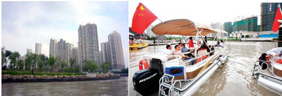
Figure 126 Suzhou Creek after the completion of waterfront promenade
