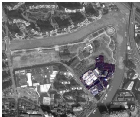
Figure 150 Aerial picture of Chunming Textile Factory. Adapted from Google Earth.
