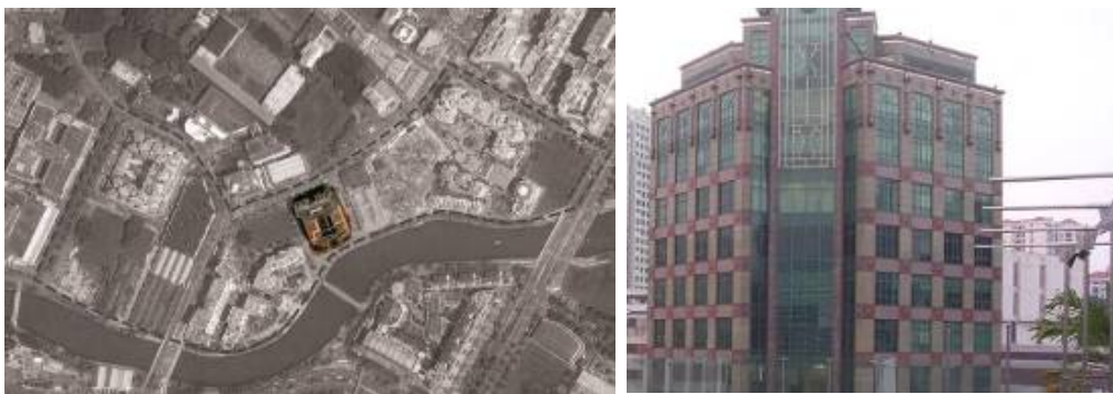
Figure 100 Riverside 48 aerial picture and photo
