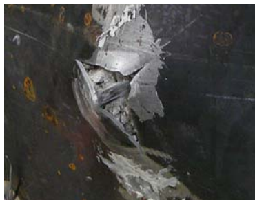
(b) Fracture point of bottom plate
