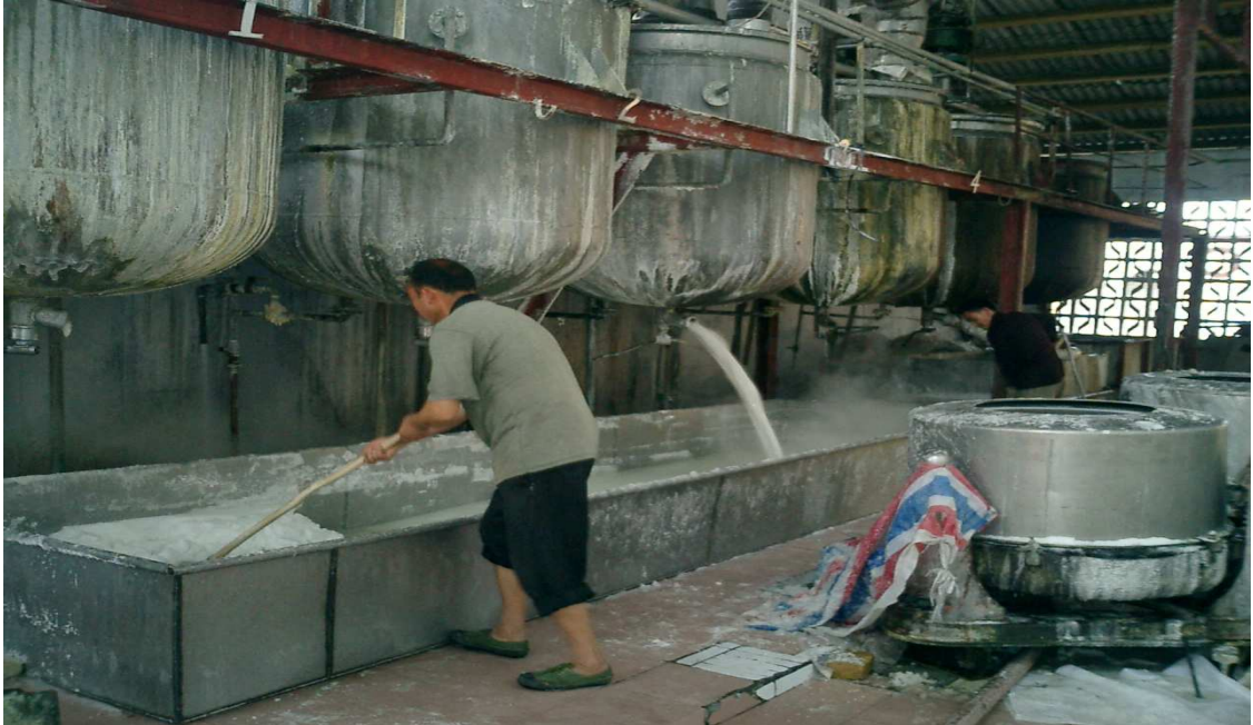
Photo 2 Sample of A Circulation Pool of a Small Scaled Phosphate Factory
