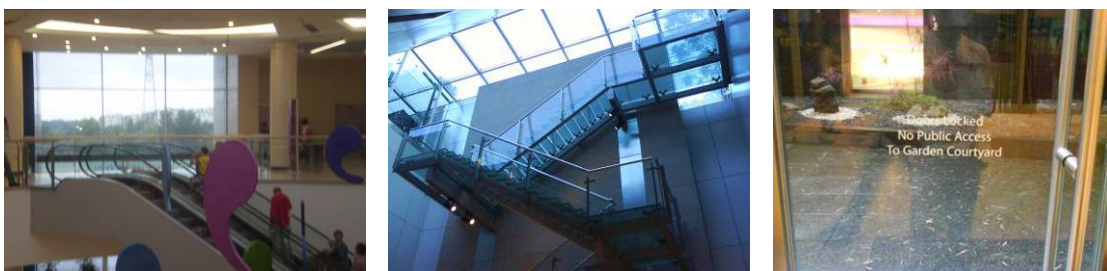
Figure 58 – Bad view: visual access to outdoor space is not necessarily pleasant, DeltaCity (left) Figure 59 – Attractive yet dysfunctional staircases, CityLink (middle) Figure 60 – Restricted access to outdoor garden, CityLink (right)
