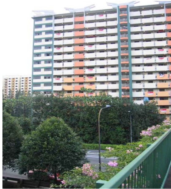
Figure 3.4 Elevation View of Block 75, near Jalan Bahagia
