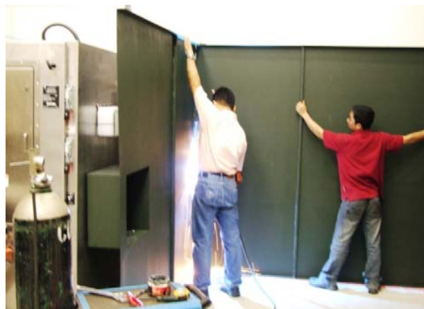
Figure 9.17 Continuous welding of the steel plates
