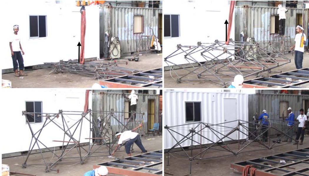
Figure 7.6. Deployment of Pyramid-Pantograph-Pyramid Structure.
