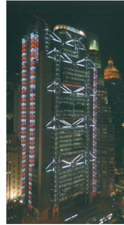
Figure 29.0 HSBC Building after implementation of Lighting Masterplan (Source: PLD magazine no.38 )
