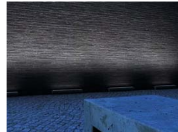
Figure 73.0 Continuous linear lighting (Source: ERCO lighting)
