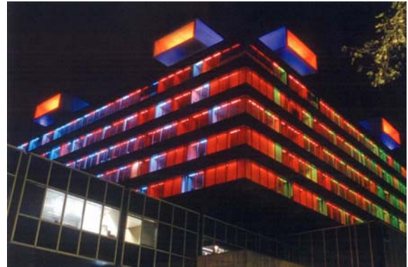
Figure 22.0. Lighting landmarks during the Festival of Lights (Source: PLD Magazine no.25)
