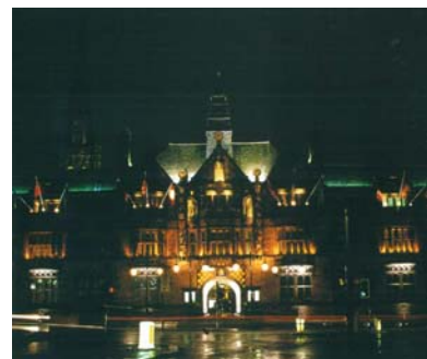
Figure 45.0 Coventry Council House (Source : PLD Magazine no.18)
