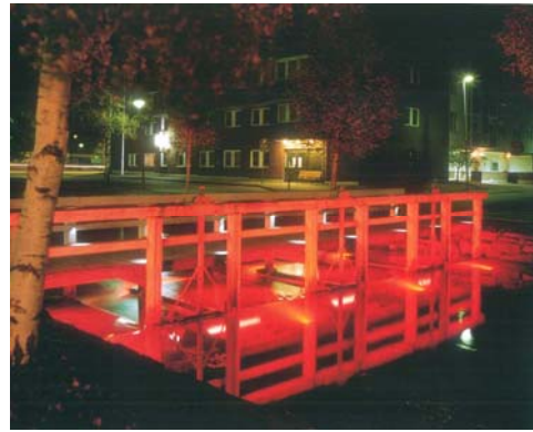
Figure 37.0 Bridge lighting (Source: PLD magazine no.18)
