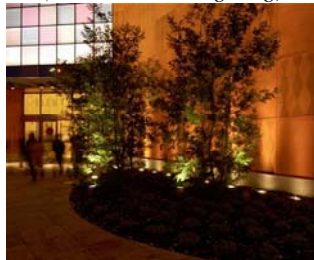
Figure 72.0 In-ground recessed up-lighter (Source: ERCO lighting)
