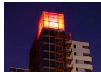
Figure 7.0 Example of installation of Colour kinetic fixture, Berkeley Homes Tower at Tabard Square London, UK ( Source: http://www.colorkinetics.com/ )
