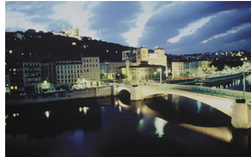
Figure 11.0. Bridge Lighting in Lyon (Source: http://www.lyon.fr/vdl/sections/en/ )
