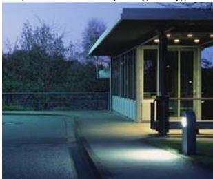
Figure 71.0 Bollard lighting (Source: ERCO lighting)
