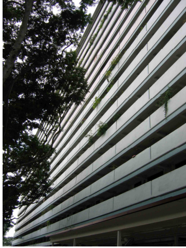
Figure 3.1 Front elevation of Building One
