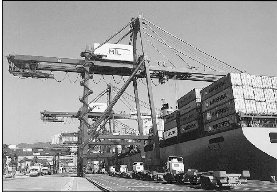
Figure 2.1 Quay Cranes in Operations (Linn et al., 2003)
