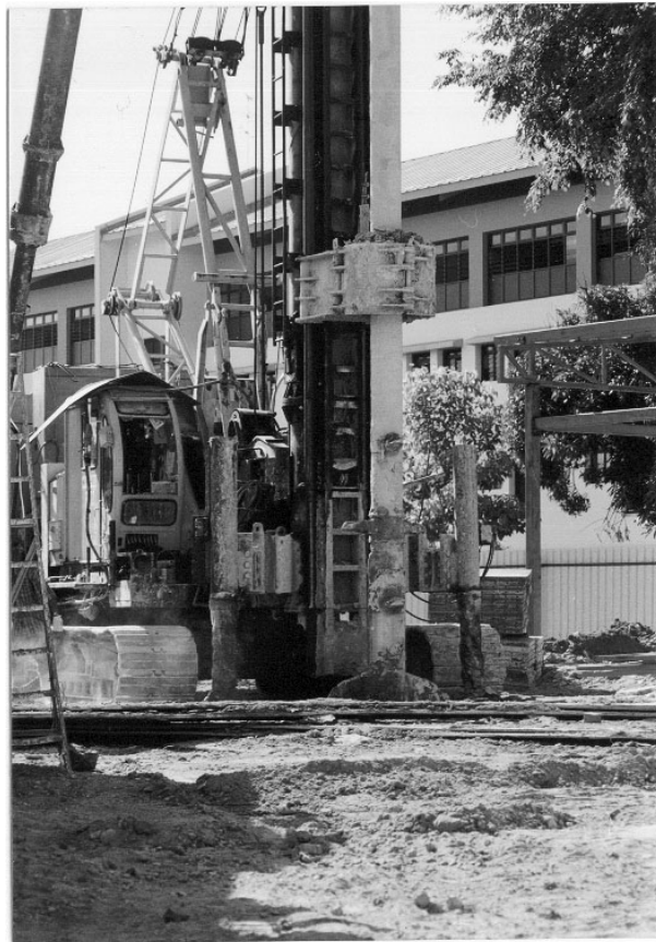
Fig. 1.2 Installation of DM column.
