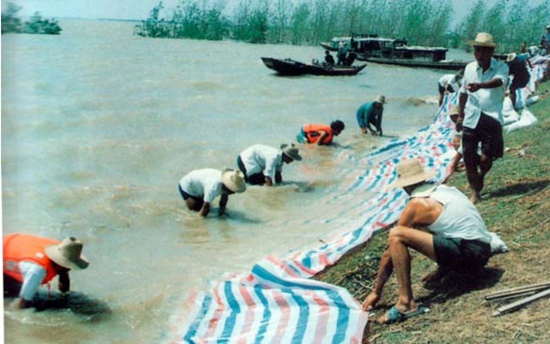
Plates 5 Overtopping of levee during flood in 1998.
