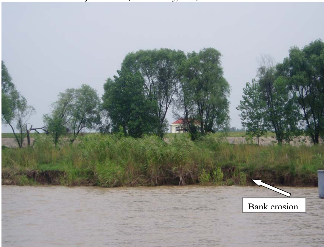
Plates 4 Bank erosion in flood season (Taken in July, 2004).
